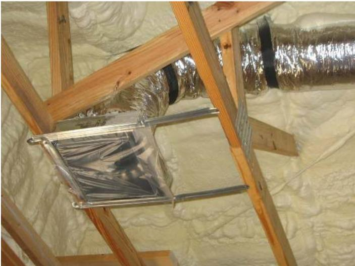
**Open-cell insulation, when qualified as an air barrier, is an effective solution to maximizing air control and minimizing related problems.**
