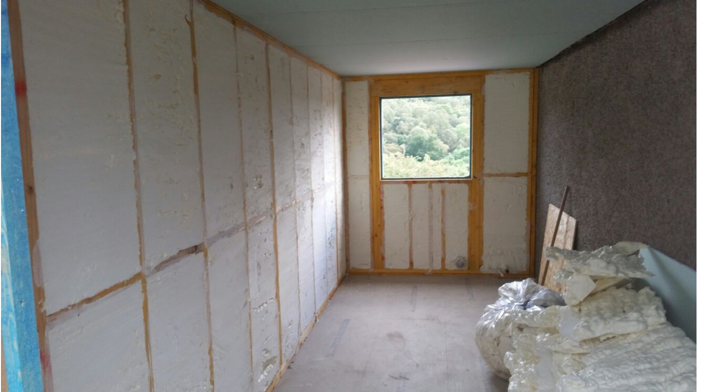
Figure 1 - the Product installed between studs prior to the application of a plasterboard lining
