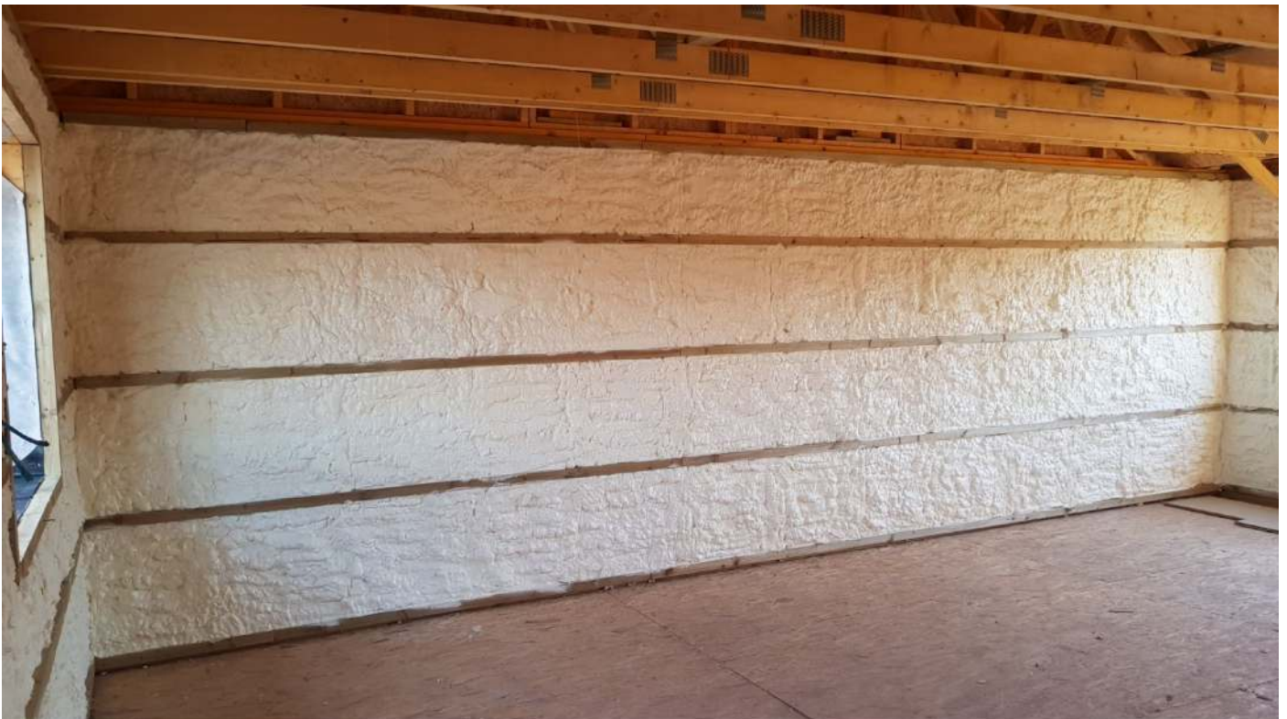
Figure 2 - the Product built up between counter battens over timber studs to minimise thermal bridging and seal the joints in the timber frame
