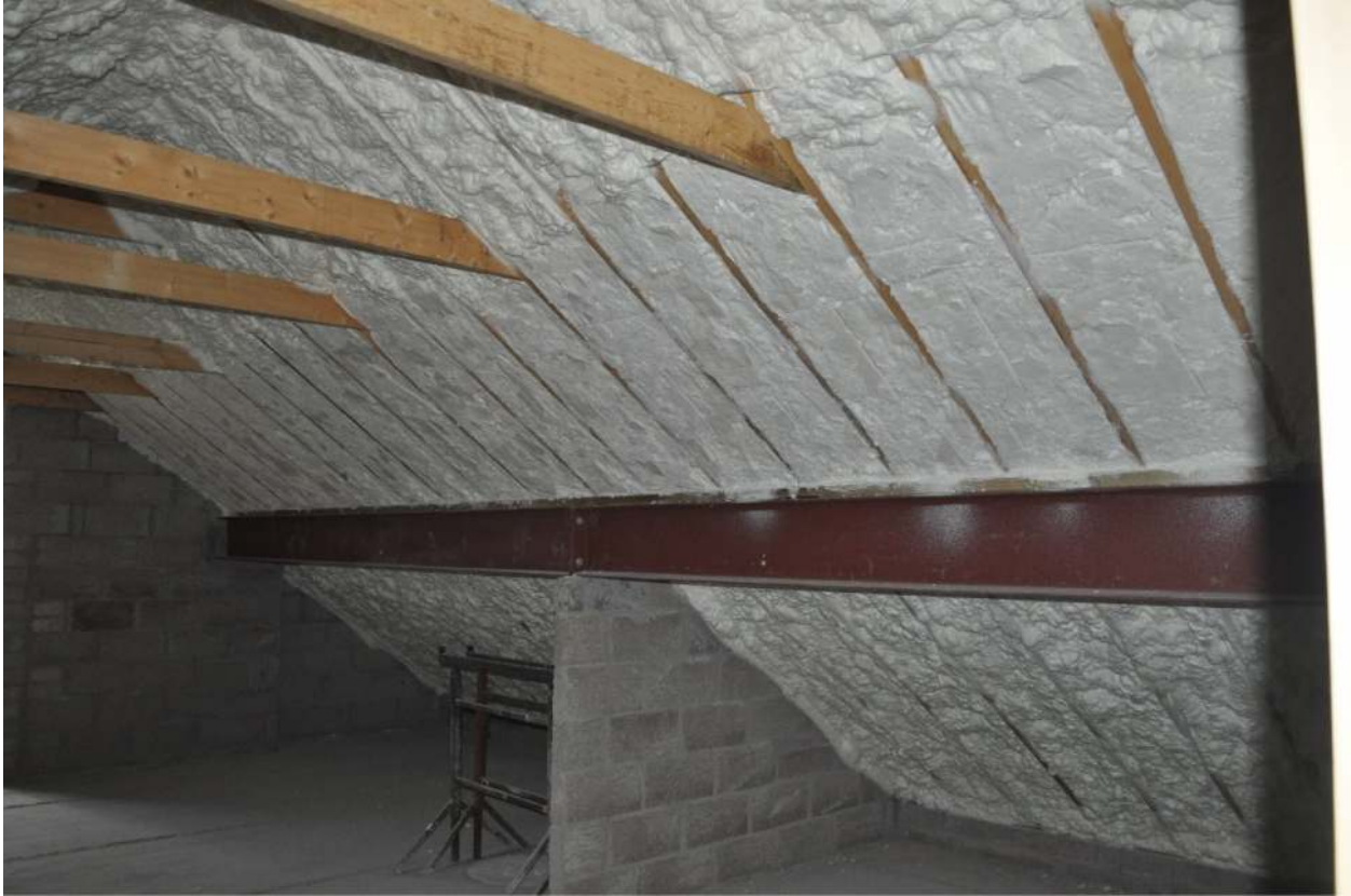
Figure 2 - Dressed back Product prior to the application of the plasterboard lining
