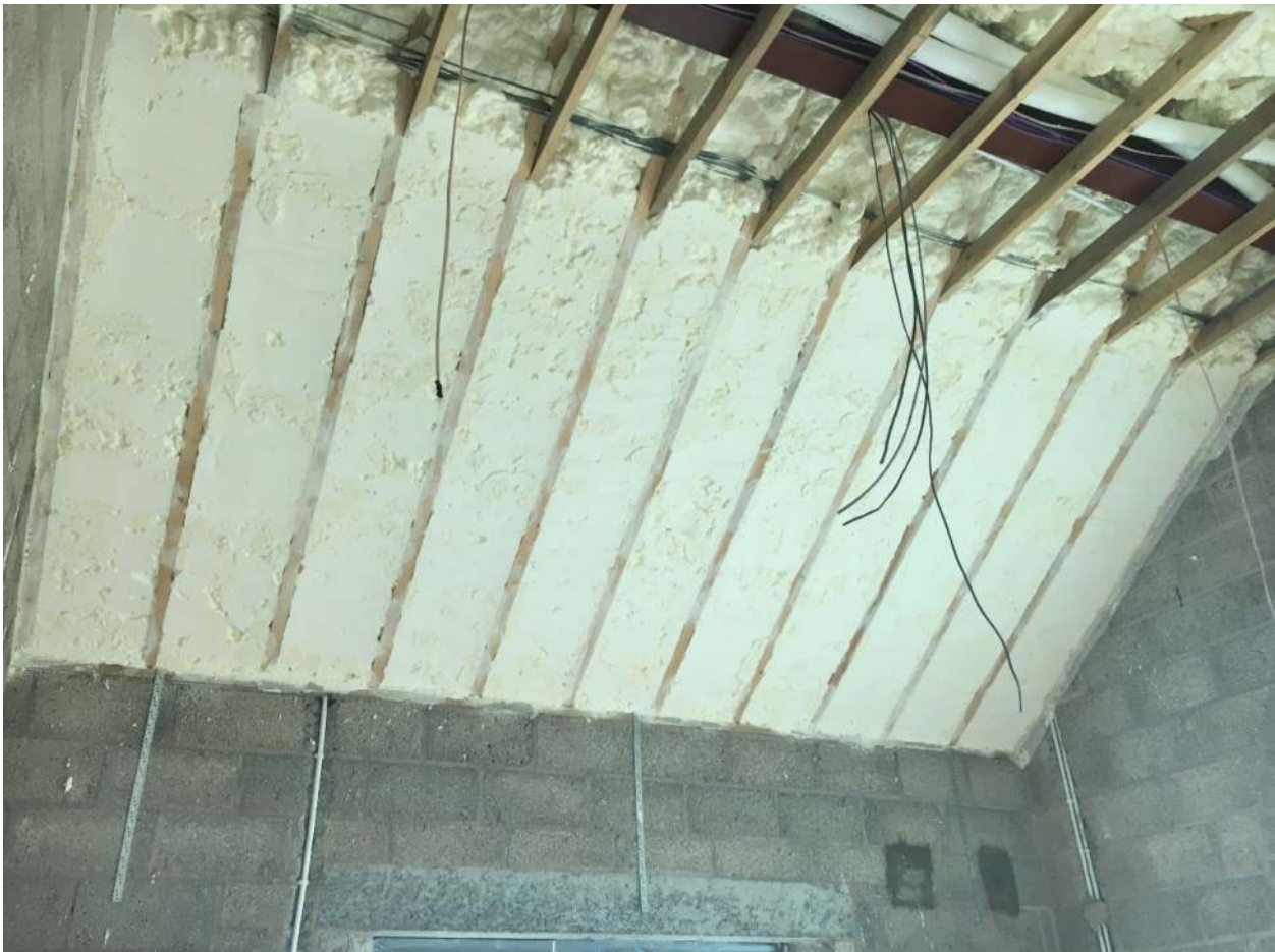
Figure 2 - Dressed back Product prior to the application of the plasterboard lining
